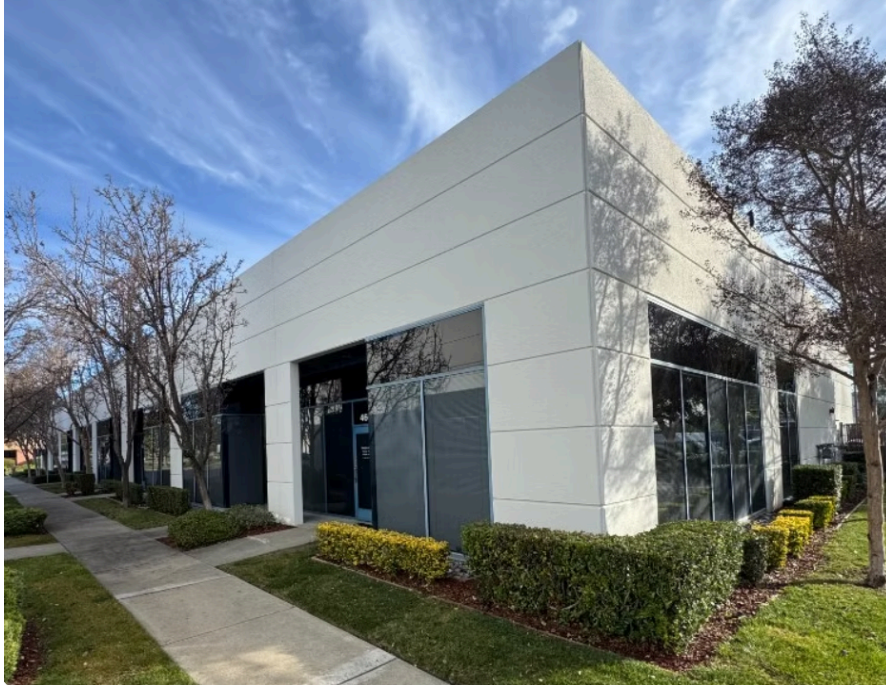
[FIGURE 1 – SpectraPower Facility, Livermore, CA]
